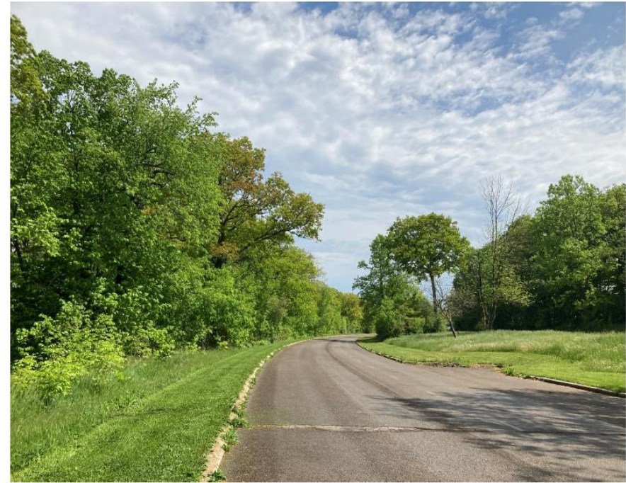
Photo 8. The closed parkway facing north.
