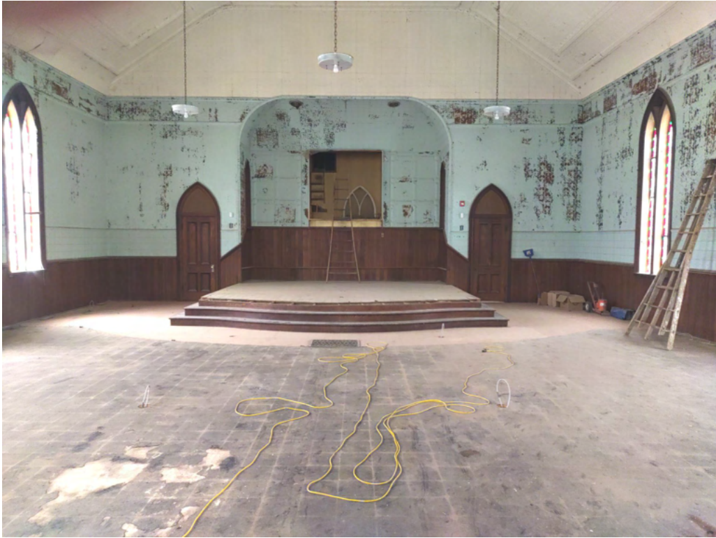
Nave, North wall:
