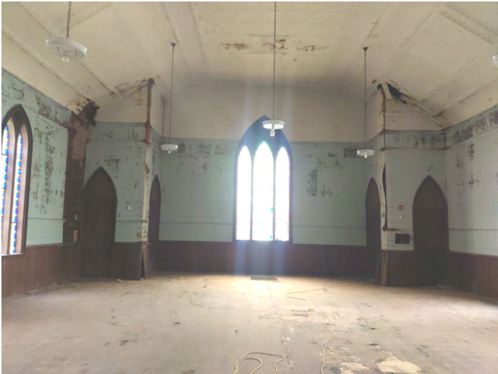
Nave, South Wall:
